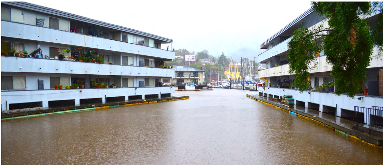
Flooding in the Canal area.
