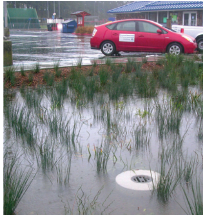
The stormwater gardens help slow, spread, and sink heavy flows.
