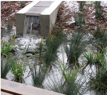
Channels bring water from the parking lot into the stormwater gardens.
