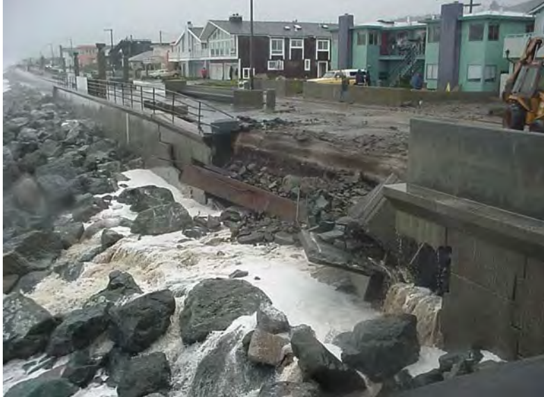
Seawall failure, Beach Boulevard, Pacifica, 2010
