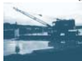
A dredger clears a creek crossing.
