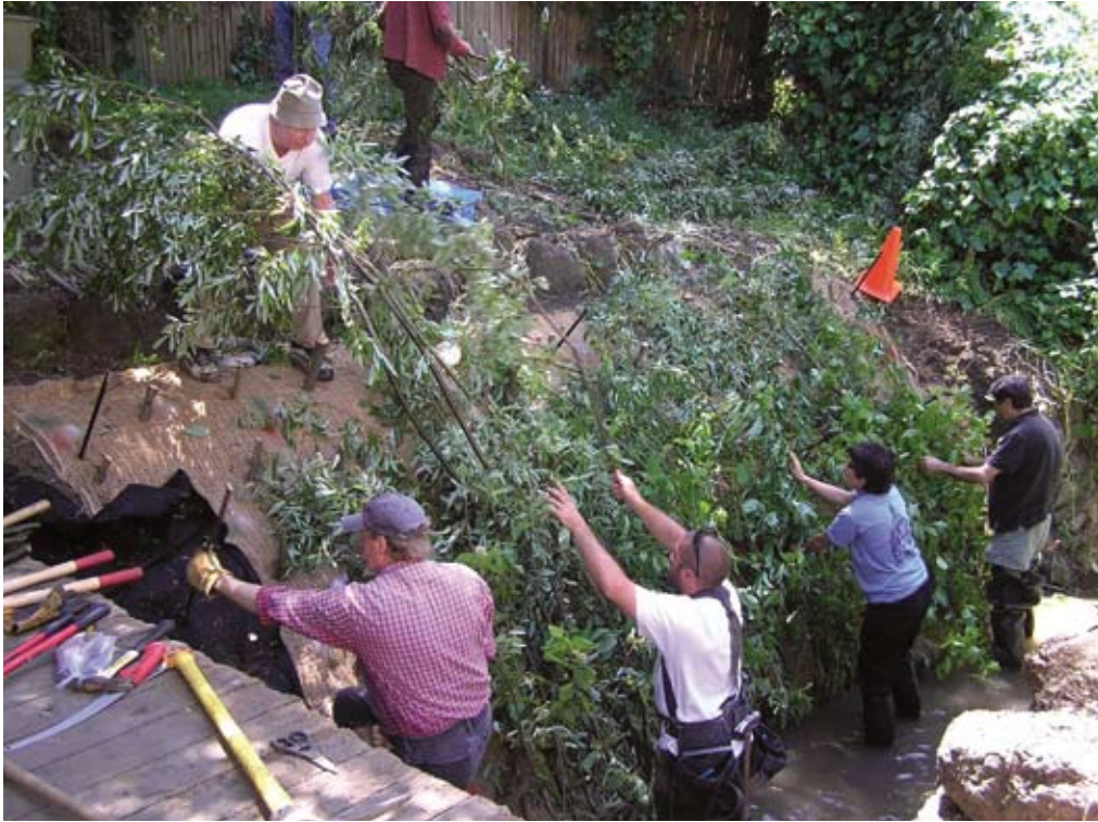
Soil bioengineering—using plants and plant parts to stabilize creek banks—is an effective alternative to riprap and provides good riparian habitat.
