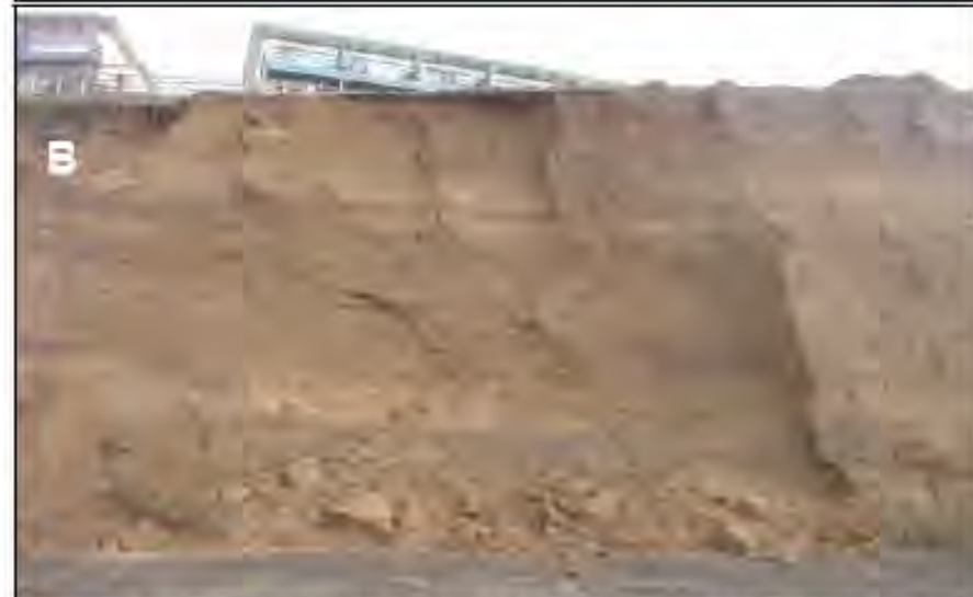
Figure 5. Schematic diagram (A) and photo (B) of moderately cemented coastal cliff failure mode. The failure surface is typically near-vertical.
