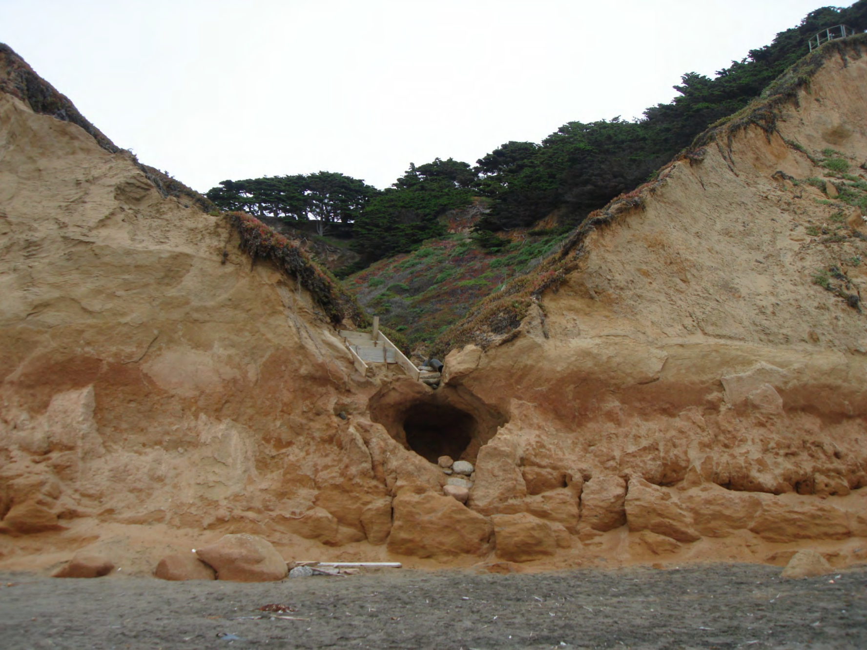
Piping ! Manor Bluffs, Pacifica Aug 2010 © Bob Battalio, 2010
