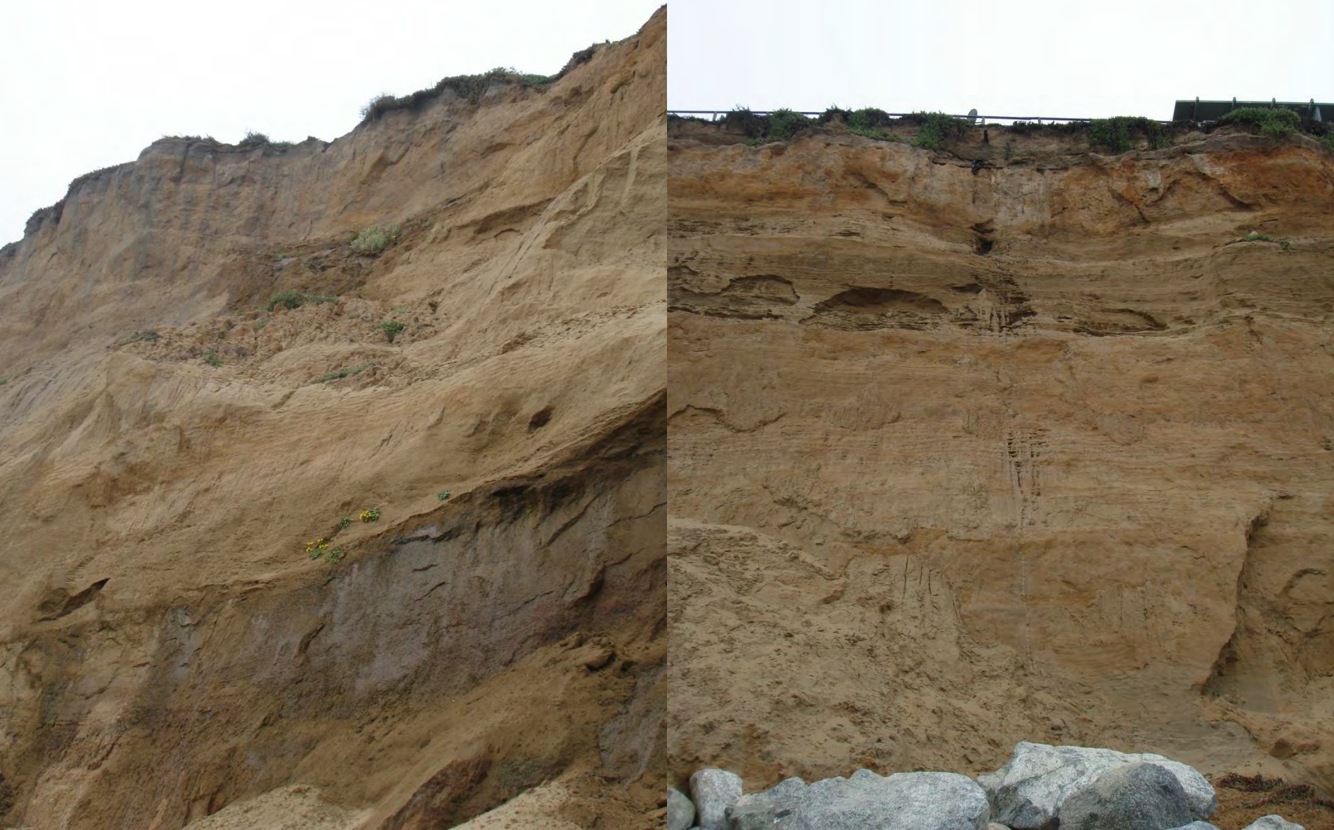
Seeps, rills and piping; Manor Bluffs, Pacifica Aug 2010 © Bob Battalio, 2010
