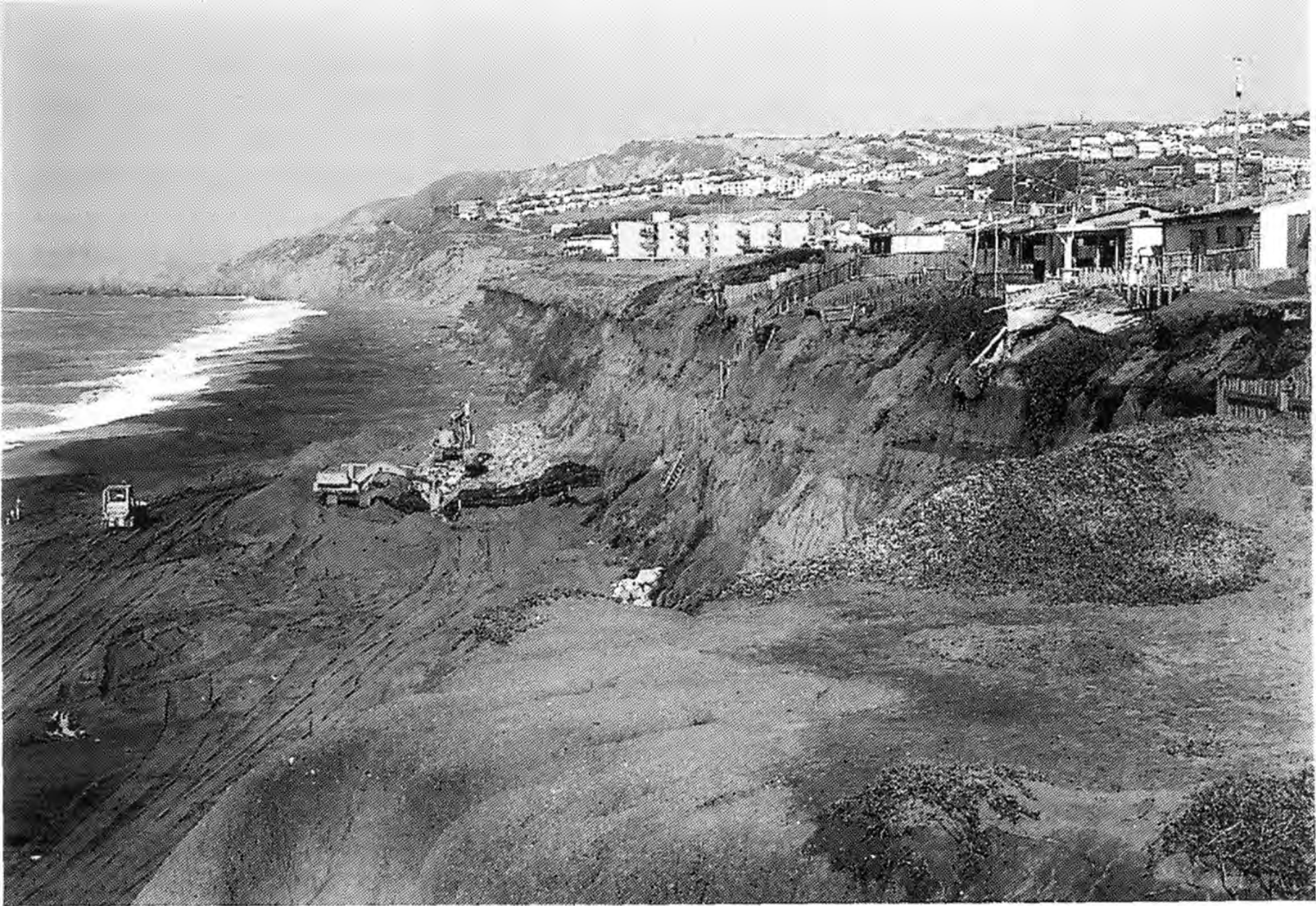
Figure 2. Pacifica bluffs in October 1983, following the last major El Niño event on the California coast, when a rock revetment was constructed.
