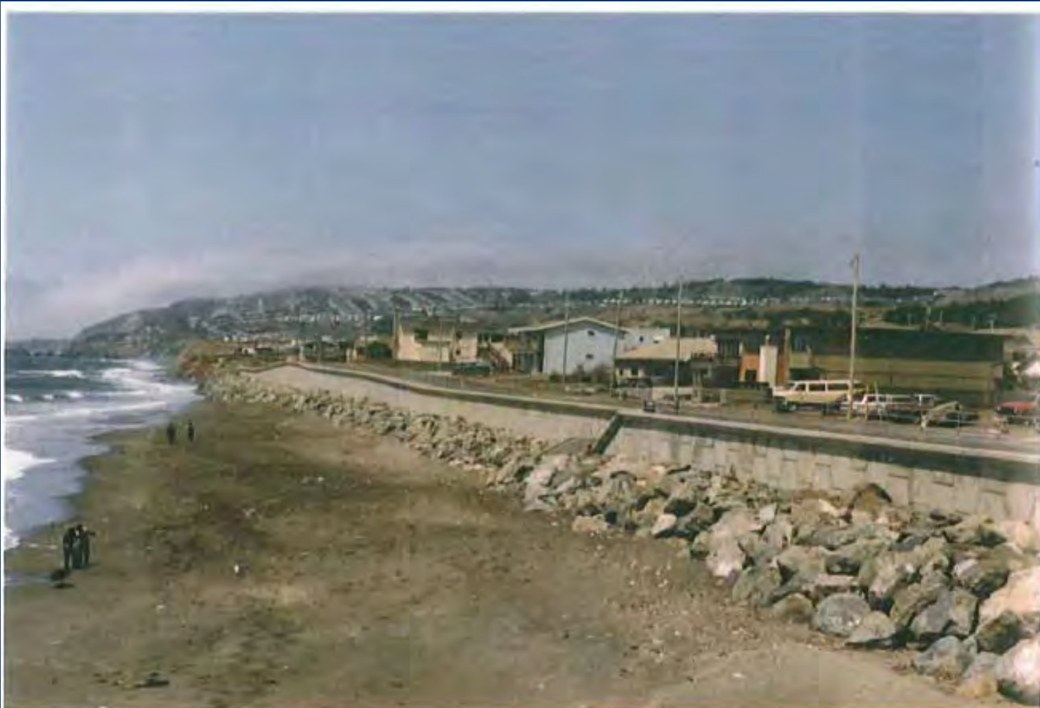
Photograph 6. Recently constructed reinforced earth seawall with armor stone toe protection. This wall extends along Beach Boulevard north of the Fishing Pier in Pacifica (August 1985).
