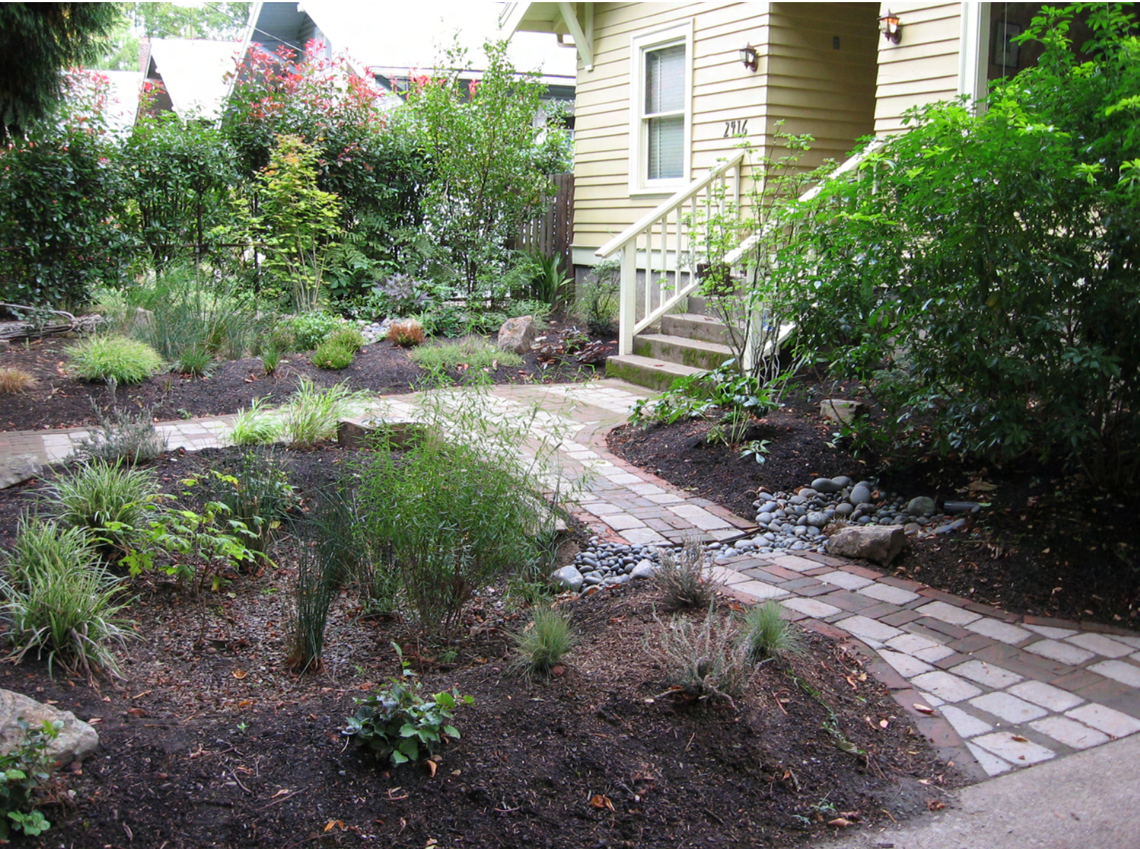
A small rain garden in the city of Portland. Photo courtesy of Portland Sustainable Stormwater Division.
