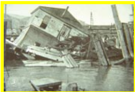
From 1919–1921, the shipworm, Teredo navalis , caused at least $2 billion (in 1992 dollars) of structural damage to maritime facilities.
